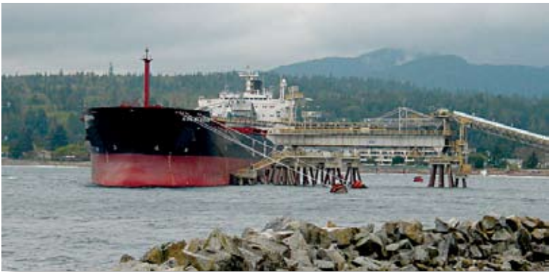
Construction Aggregates' loading dock, Sechelt - Edwin Huber photo
